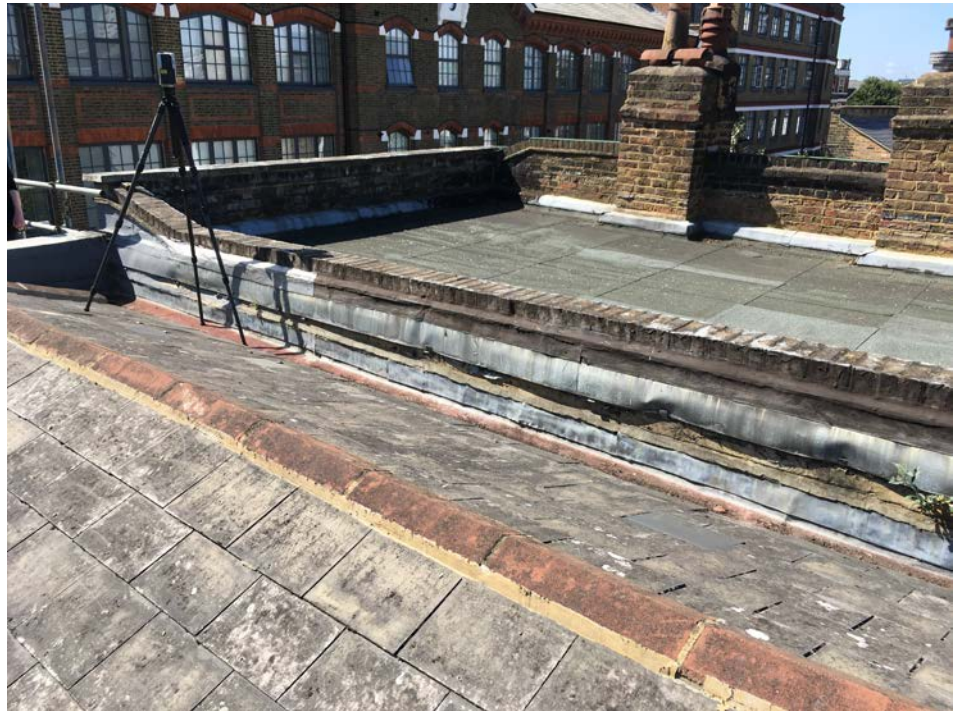
Flat roof to No. 22 Anglers Lane
