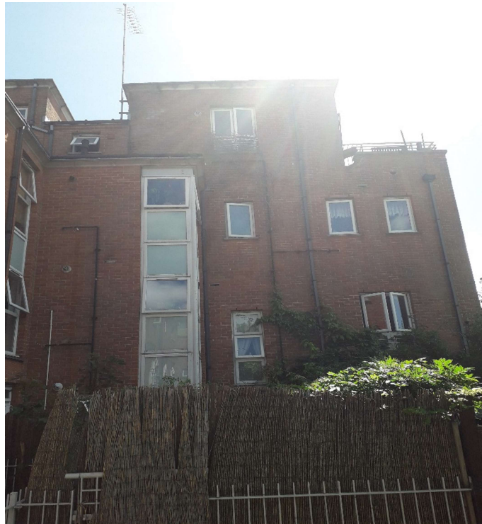
Photograph 05 – North Elevation (Rear)
