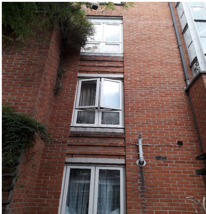
Photograph 02 - South Elevation - Timber windows
