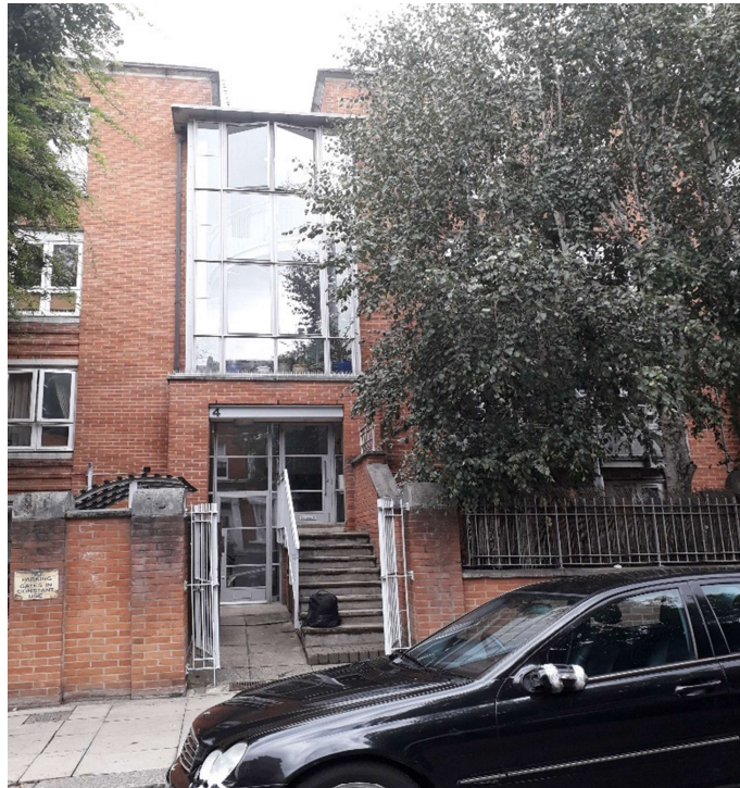
Photograph 01 - South Elevation (Front)
