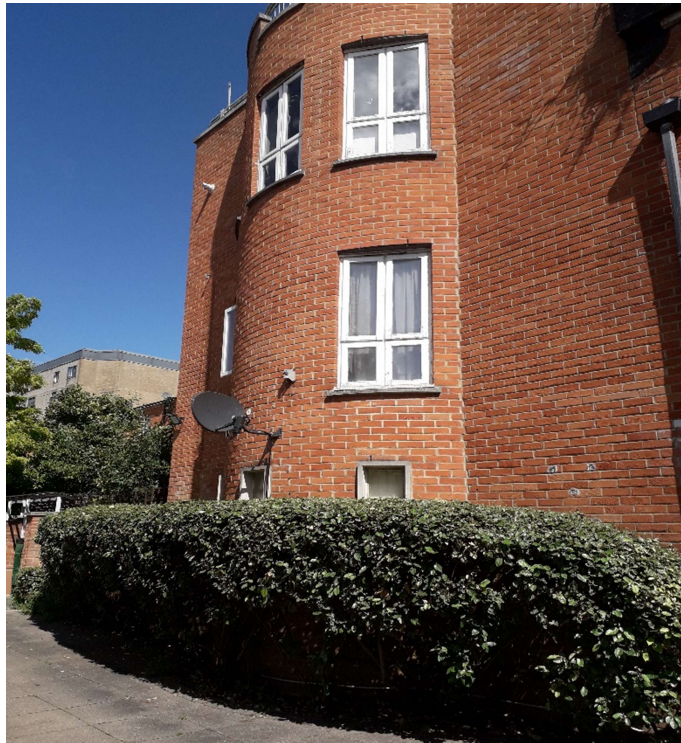
Photograph 04 – West Elevation (Side)
