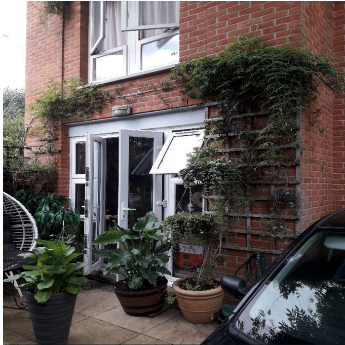
Photograph 03 – Flat A, Doors replaced with PVCU
