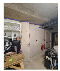
New cable to be installed alongside the path of the existing cable along the roof as indicated above, where it will join the cable on the existing trunking and enter into the communications room.
