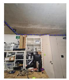
New cable to be installed alongside the path of the existing cable along the roof as indicated above, before turning at the wall and running past the communications room.
