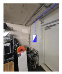
The new cable will run into a new BFP that will be installed along the wall, with the cable running back along the same path where it will then double back across the top of the door as shown above.
