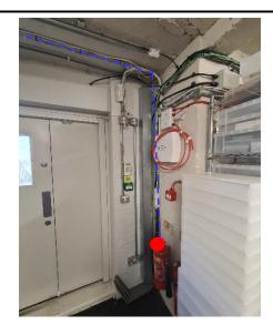
New cable will enter inside the building via the existing duct, and then run up the door passing to the other side of the door.
