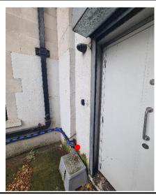
New cable to be installed along the existing route, following underneath the pipe as marked above, where it will then run through the existing duct in the wall as shown. Note: As this building is part of a category 2 heritage site, the cable may have to run up to the ceiling on the opposite side of this wall (as shown in square 7)
