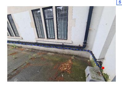
New cable to be installed along the existing route, following underneath the pipe as marked above, where it will then run through the existing duct in the wall as shown.
