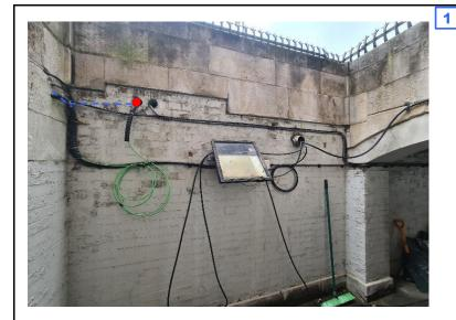
New cable to be installed via the existing duct along the wall, and follow the existing cable as shown above.
