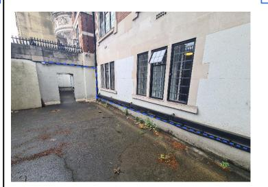
New cable to be installed along the existing route, following underneath the pipe as marked above.
