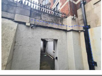
New cable to be installed via the existing duct as marked above, running along the wall and down via the pipe.
