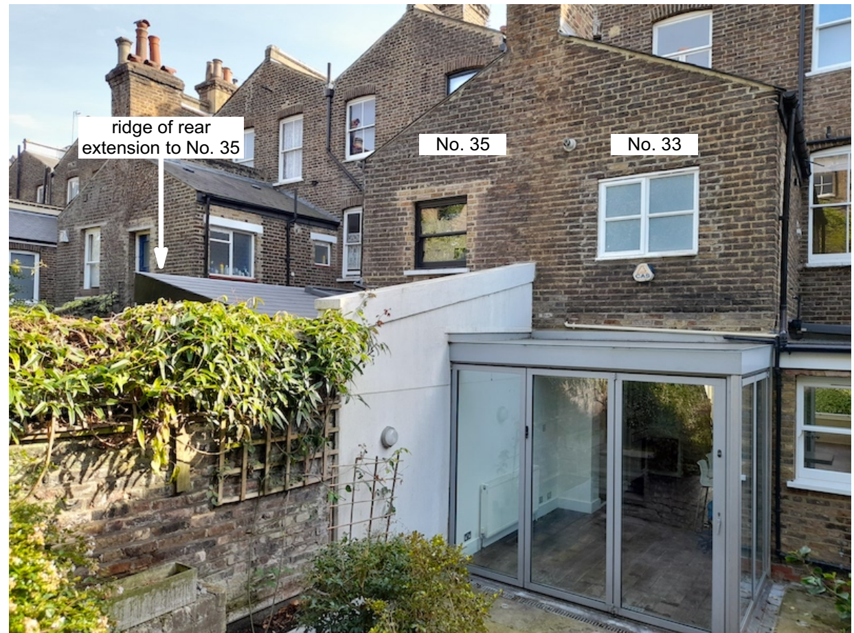
fig. 08 - The tall parapet party wall between No. 33 and No. 35 with the ridge line of the existing extension to No. 35 just visible over the garden wall.
