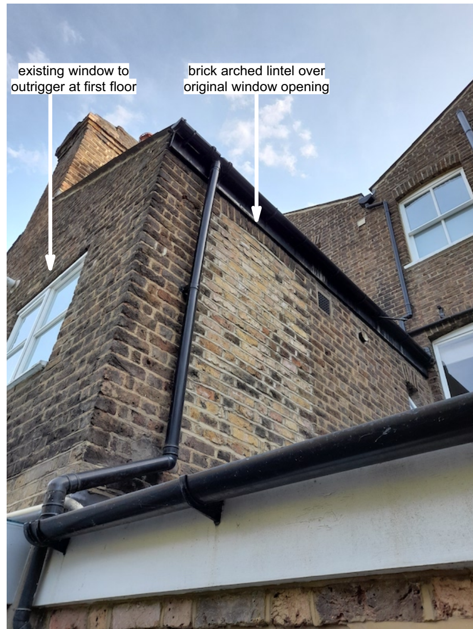
fig. 12 - The original window to the side of the outrigger at first floor has been infilled with brickwork, it is proposed to reinstate this window.
