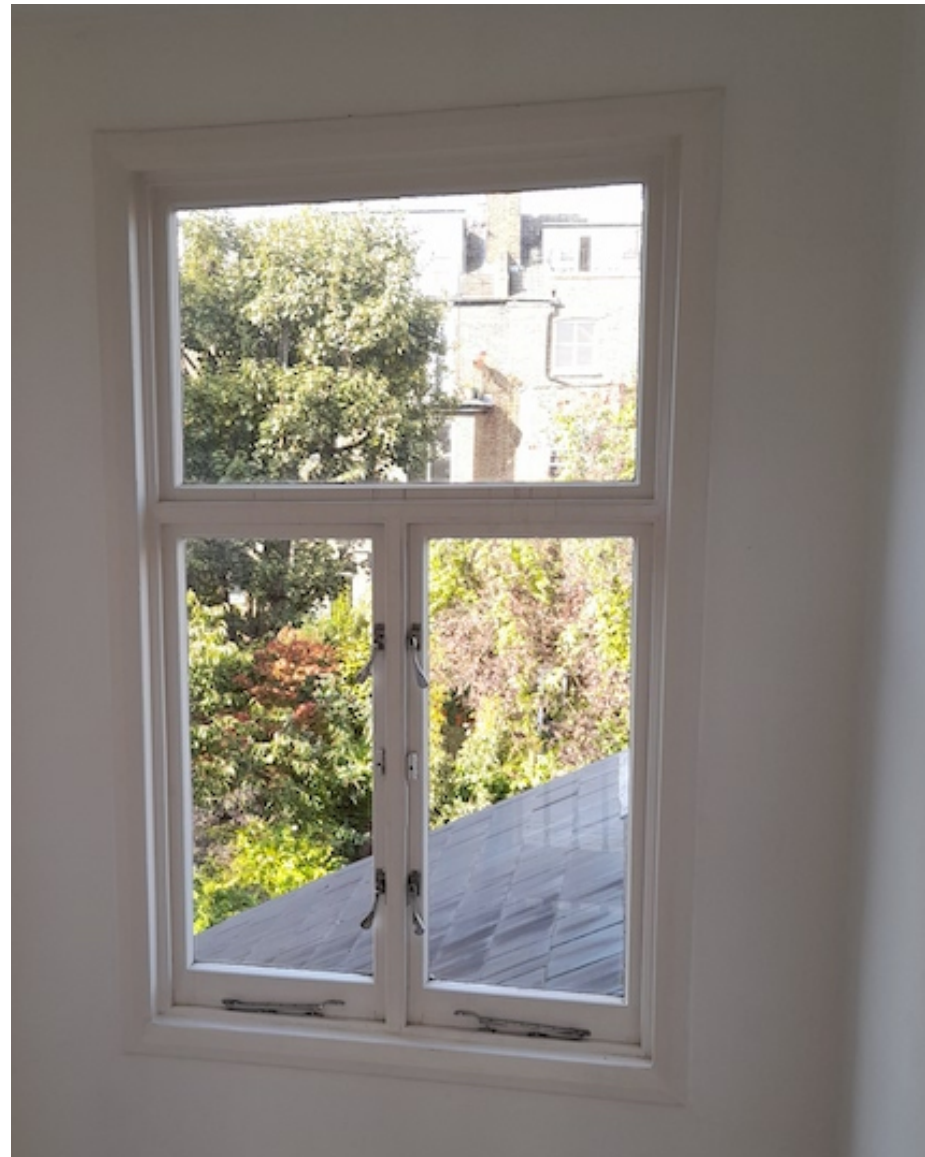
fig. 13 - The existing window at the top of the stairs is a casement window which is not in-keeping with the traditional sash windows found elsewhere. It is proposed to replace this window with a traditional timber framed sash window with double glazing.
