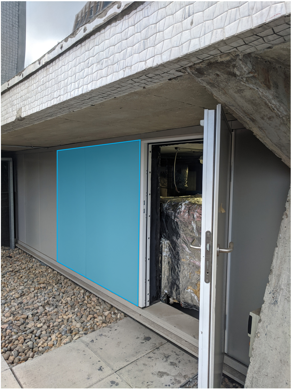
Indicative position (marked in blue) of louvres on existing plant room facade at second floor level Centre Point House (east side)
