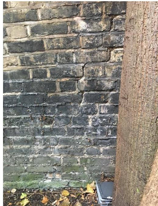
Figure 4: T6 Lime close to boundary wall with stepped cracking.
