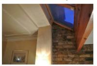
It is apparent that there has been downward and rotational movement of the rear single storey extension relative to the rear elevation of the main building resulting in a vertical tapering crack to the left hand flank wall at the junction between the structures.
