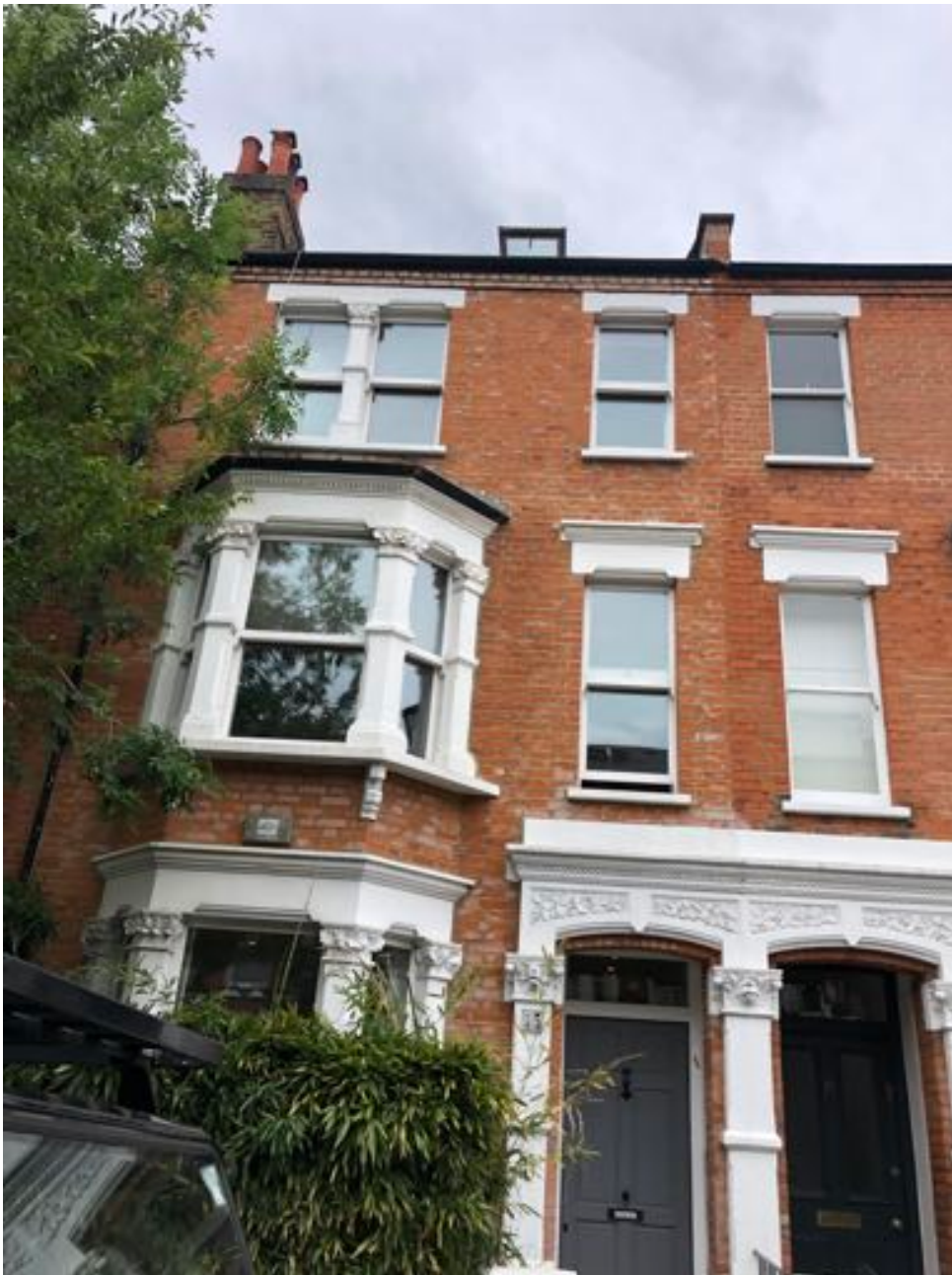
Photograph from Mackeson Road
