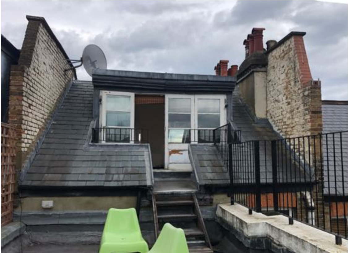
Photograph of existing loft extension
