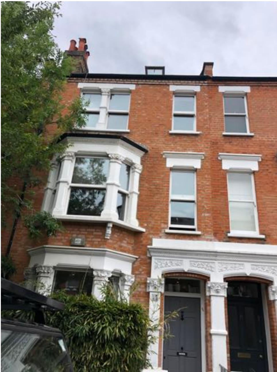
Photograph from Mackeson Road
