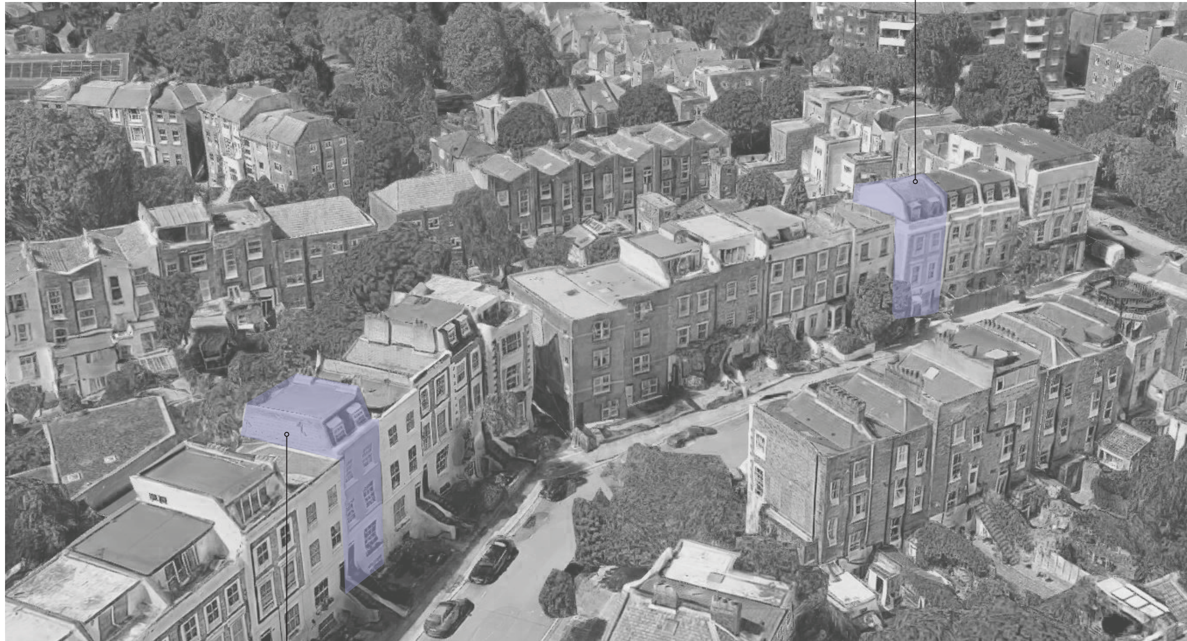
135 Torriano Avenue Demonstration of a traditional mansard roof extension
