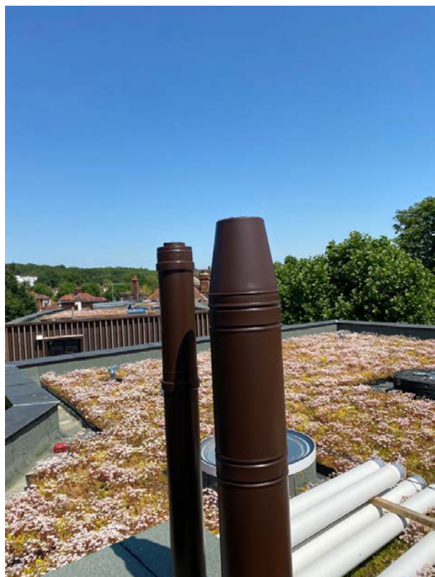
Figure 5 - Photograph of the flue painted matt bronze.
