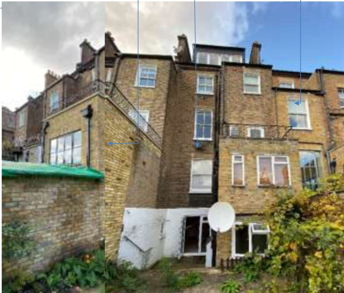
Existing Main House rear elevations to nos. 41, 43 & 45
