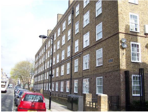
Figure 12: Walker House, North Block
