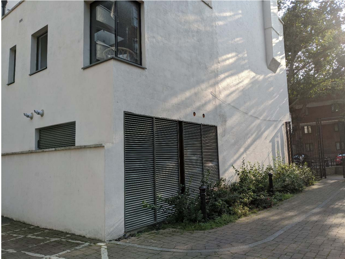
Rear Extension and Flank Wall to The Cock Tavern
