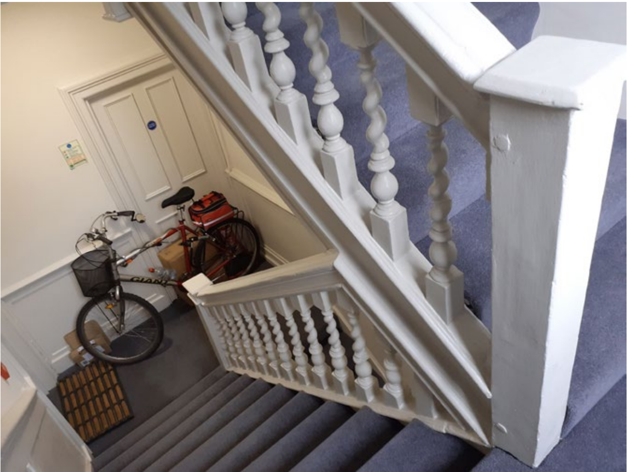
Plate 1 Early Eighteenth Century Stair (Insalls)
