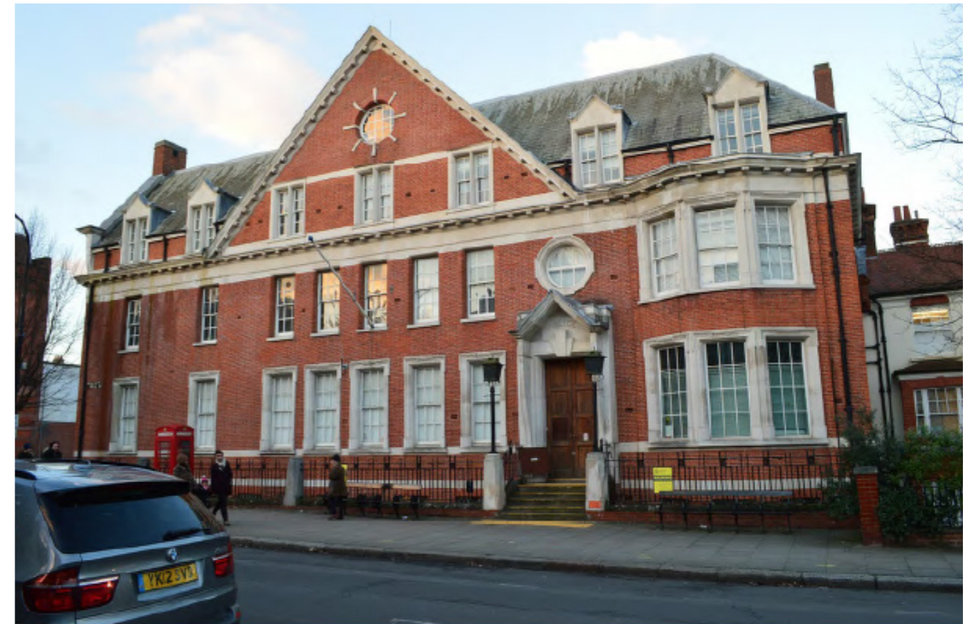
General view of the Rosslyn Hill front of the police station, showing the main entrance; part of the street front of No. 26 is just visible to the extreme right
