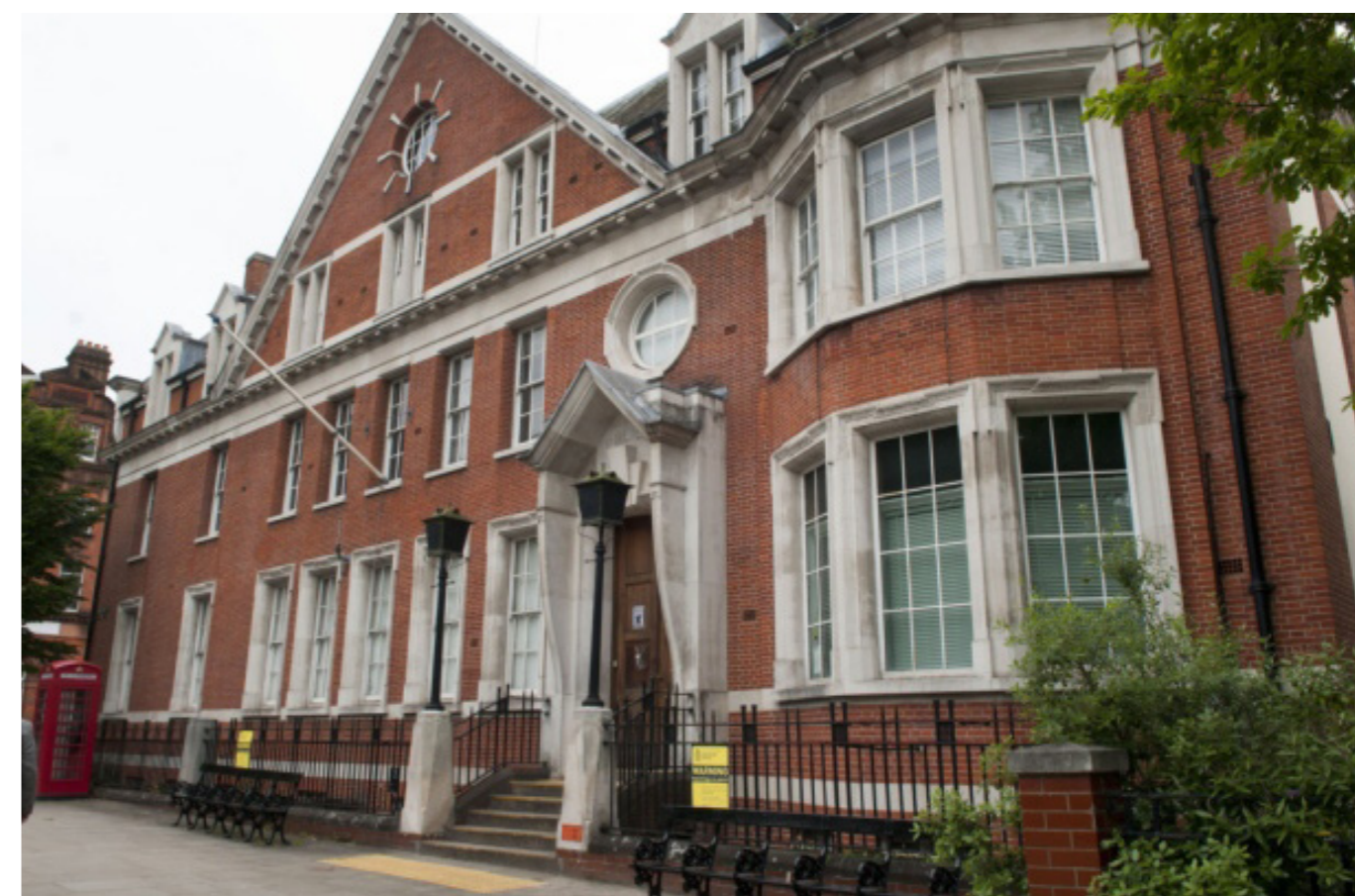
General view of the Rosslyn Hill front of the police station, showing the main entrance
