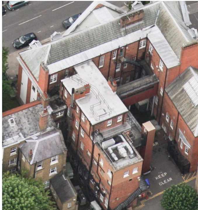
NEW STAIR TO POLICE STATION
