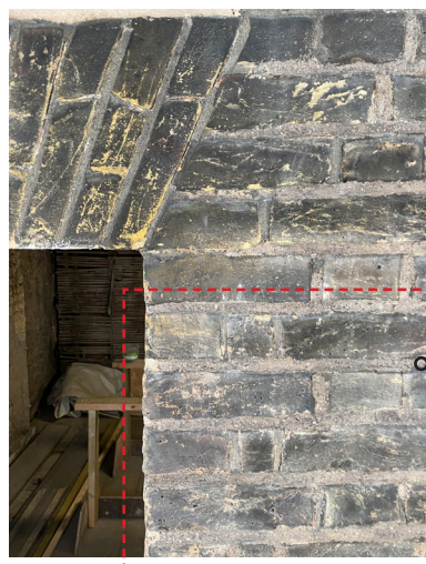
Sample area - method as image left, with pointing subsequently sooted down to soften appearance and unify existing and new
