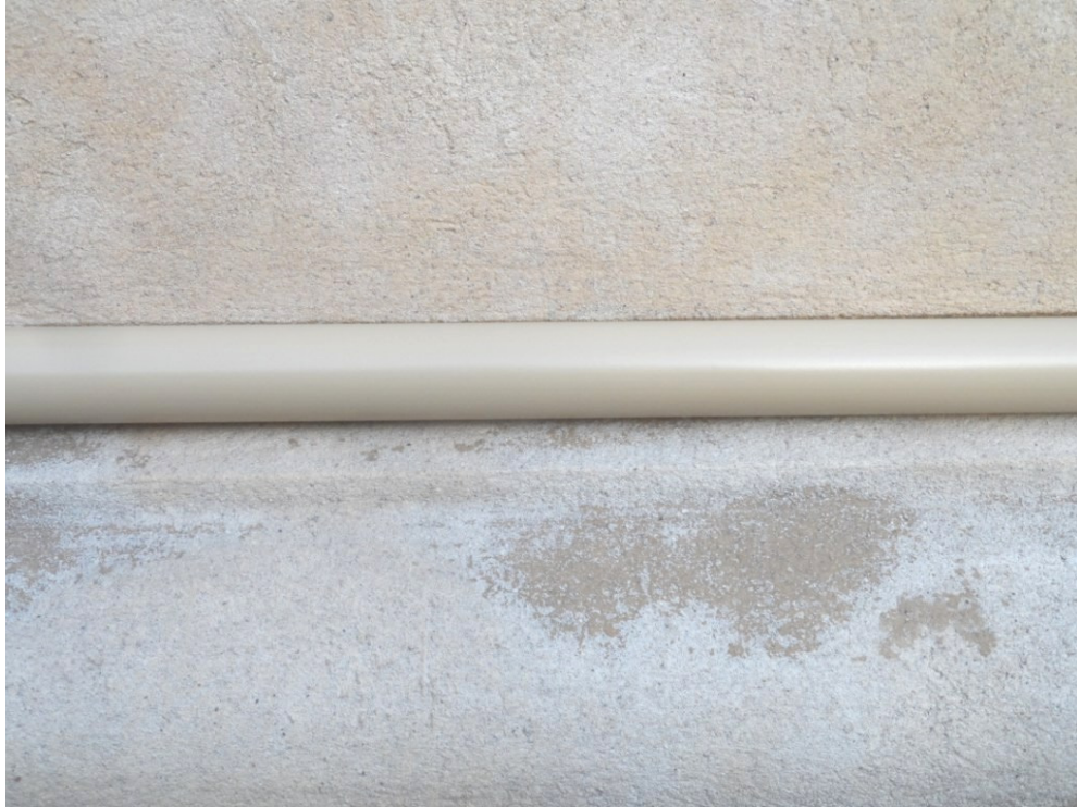
Figure 2 MOCK UP OF PROPOSED RAL 1001 CONDUIT TO SIDE ELEVATION
