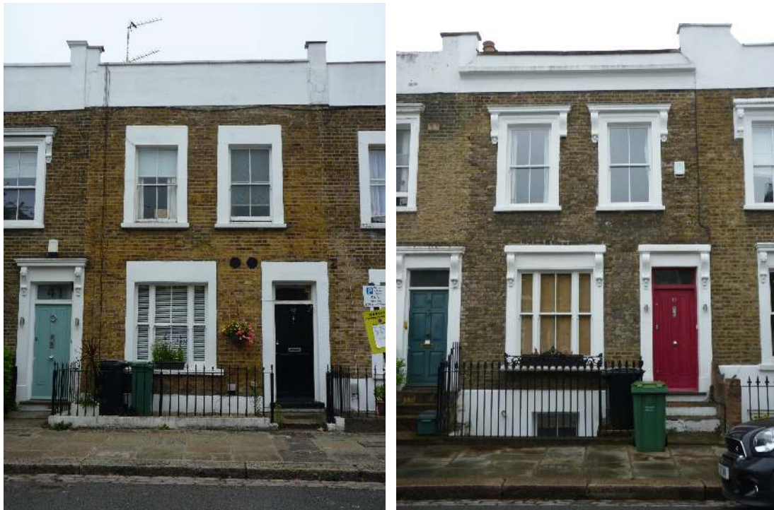
No. 42 compared with a neighbouring property retaining decorative stucco details
