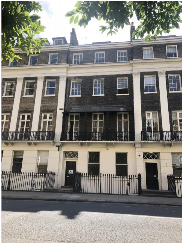
Figure 2: Photograph of the site (Source: Author's own)
