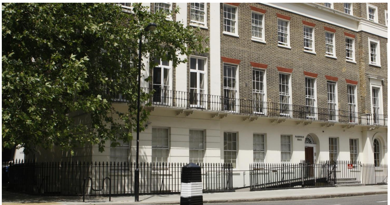
Figure 8: Passfield Hall, 1-7 Endsleigh Place (source: Ise.ac.uk, accessed 21 August 2020)
