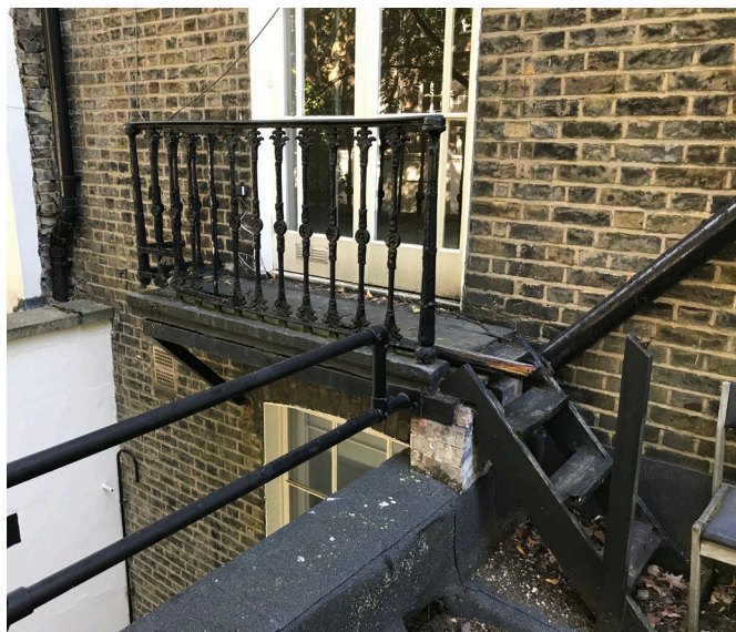
Photograph of current Juliette balcony WITH modern timber alterations and metal balustrade to parapet
