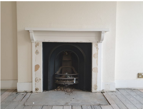
Plain painted timber on third floor with overboarding removed
