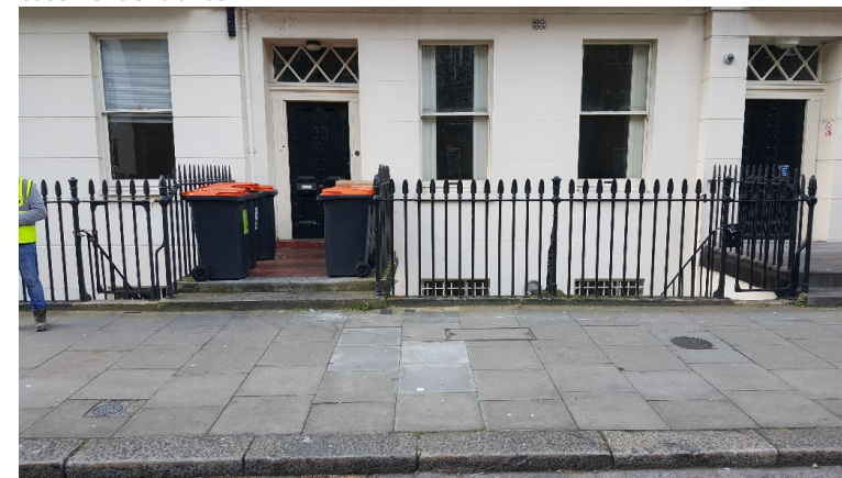
Existing iron railings and differing levels to be altered to provide wheelchair access
