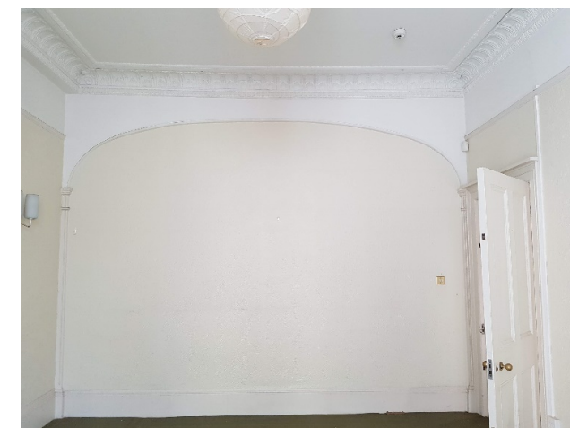
Photograph of the infilled arched opening in the wall dividing the two reception rooms on the First Floor
