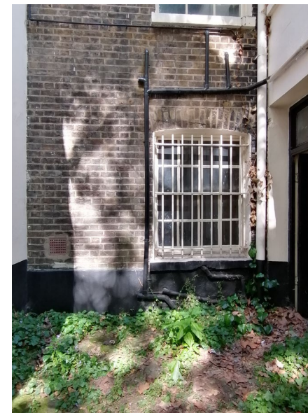
Photograph of existing modern air brick in rear elevation and drawing showing how the new extract fan will be disguised and use the existing opening
