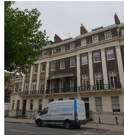
No. 13-15 Endsleigh Street, showing 2 storey addition
