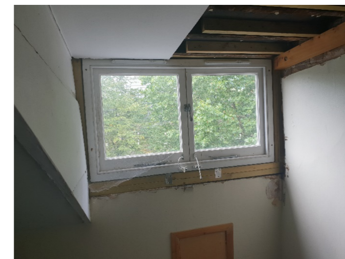
Recent structural and waterproofing repairs to dormer roof
