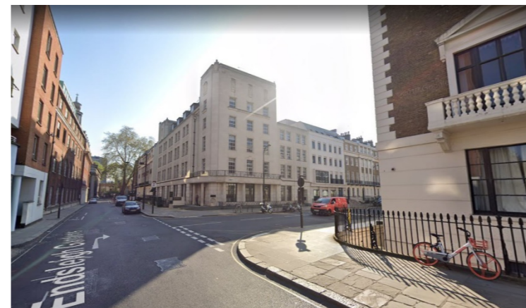
Edge of Leslie Forster House – Bentham House – corner of no. 9-14 Endsleigh Gardens
