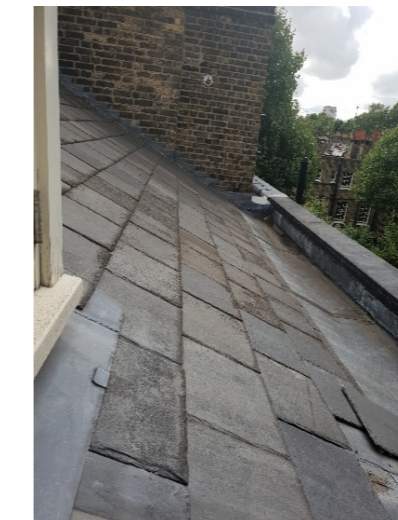
Main Roof and parapet gutter
