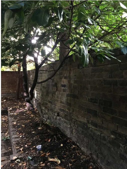
Figure 1: T1 and bulging boundary wall.
