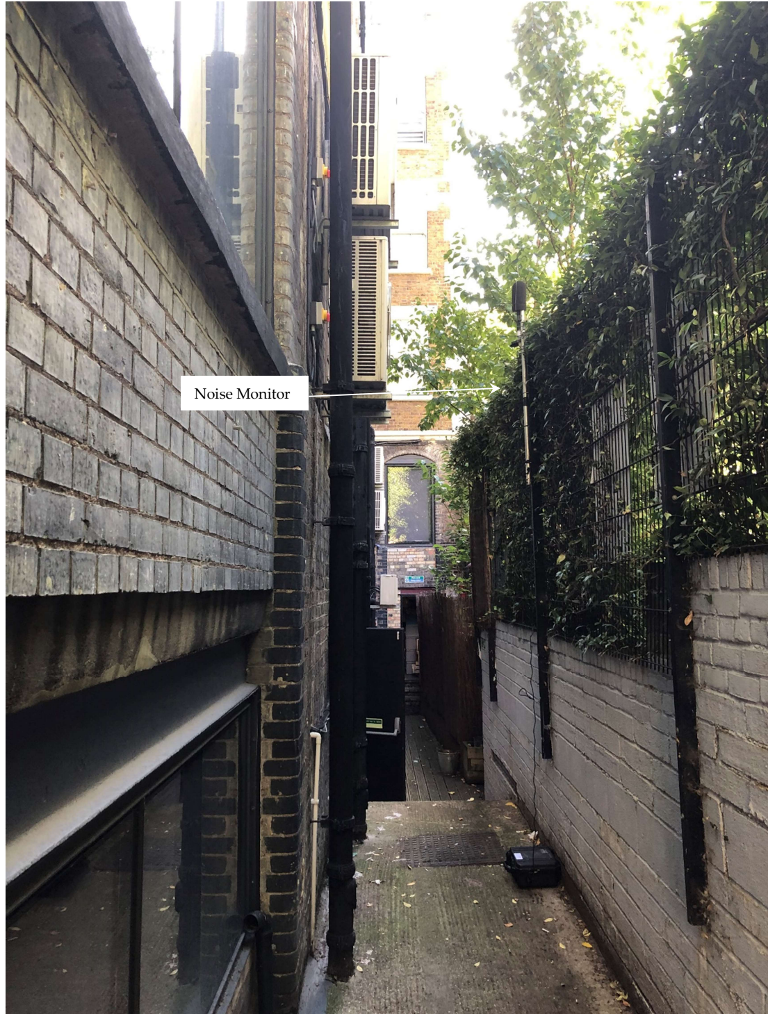
Figure A2: Noise Monitoring Equipment at rear of 1 Rosebery Avenue
