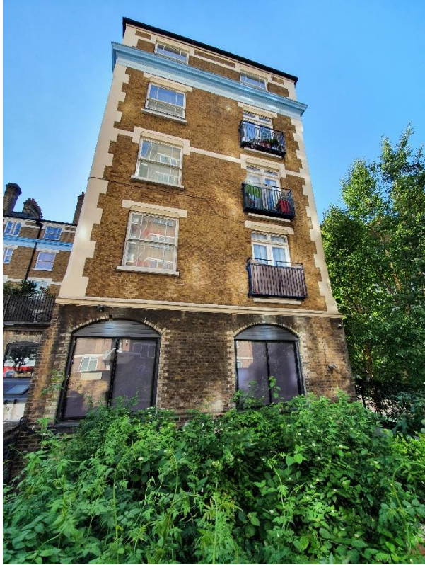
Photograph 10 – East elevation part 1
