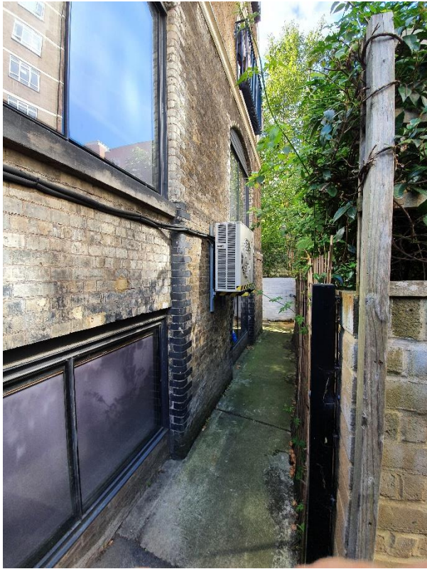
Photograph 16 – East elevation part 1
