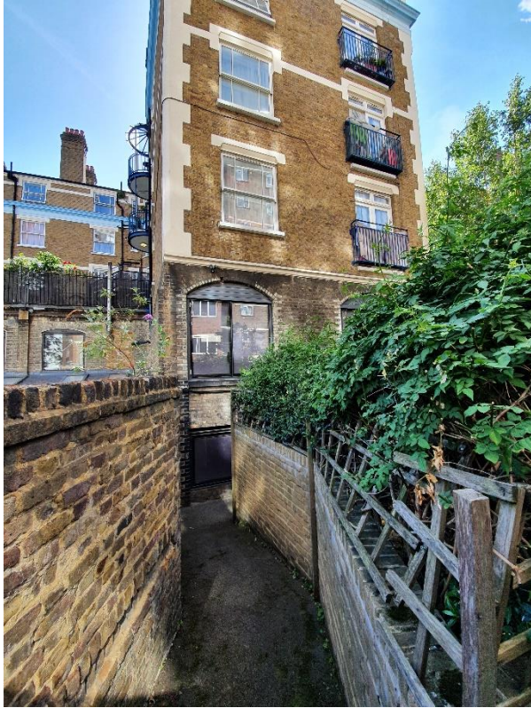
Photograph 13 – East elevation part 1
