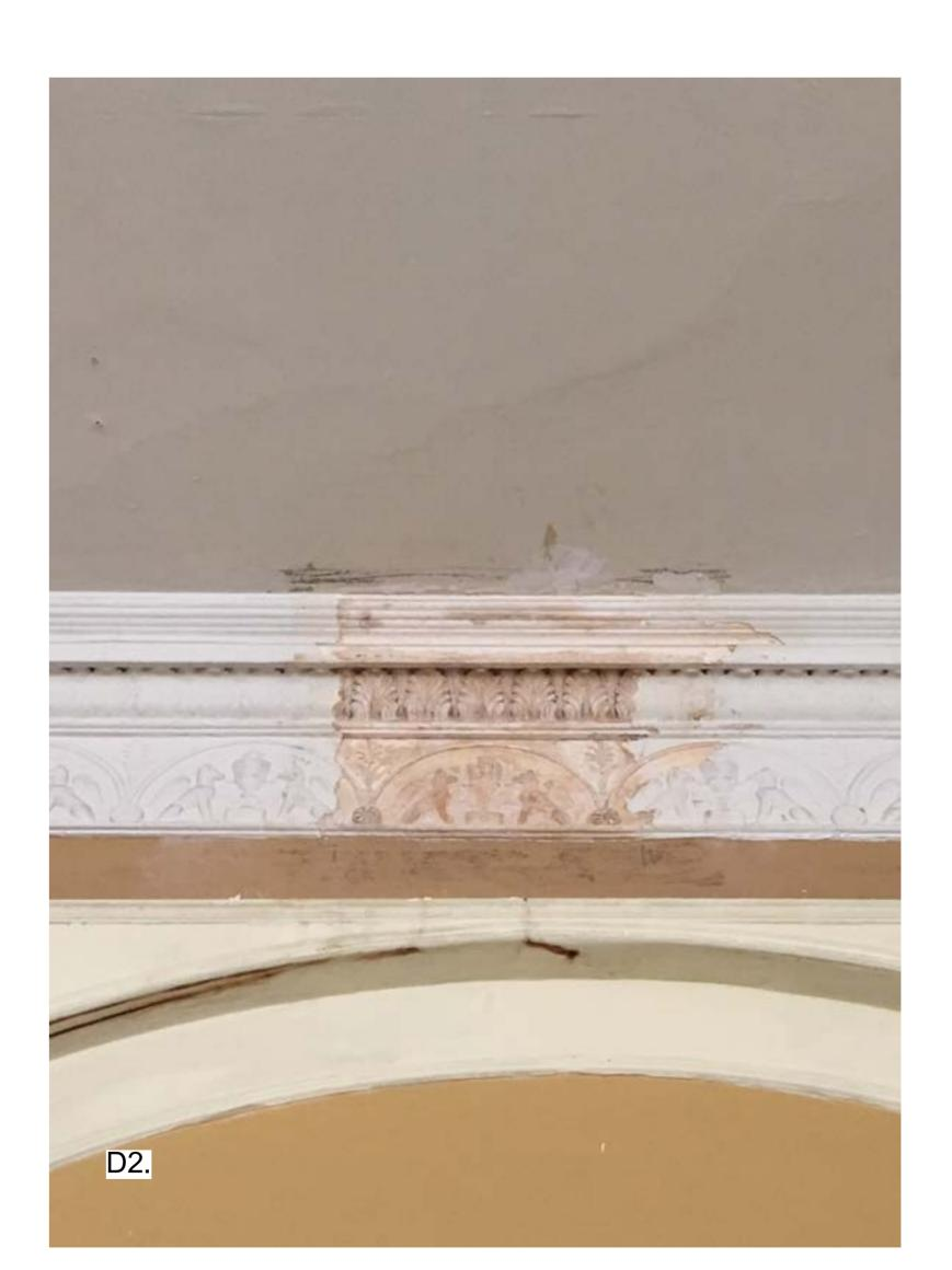
PLASTERWORK REPAIR SAMPLES (all carried out as part of approved opening up and sample works of April 2020)
