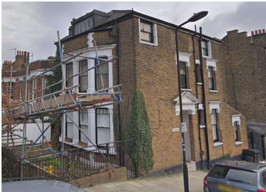
Photo 1: Gondar Cottage, Gondar Gardens
