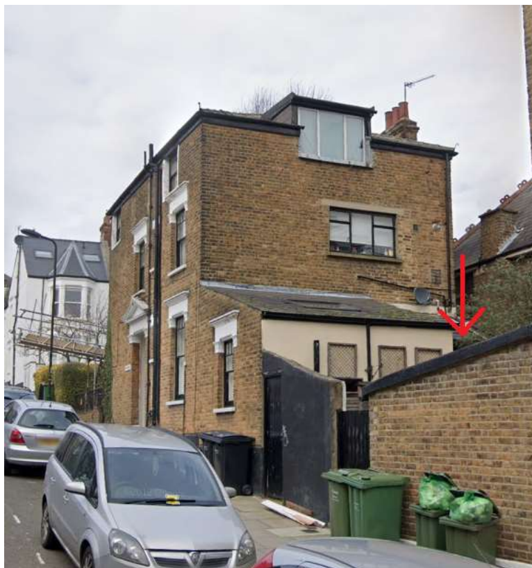
Photo 2: Rear of Gondar Cottage with location of ground floor test window marked
