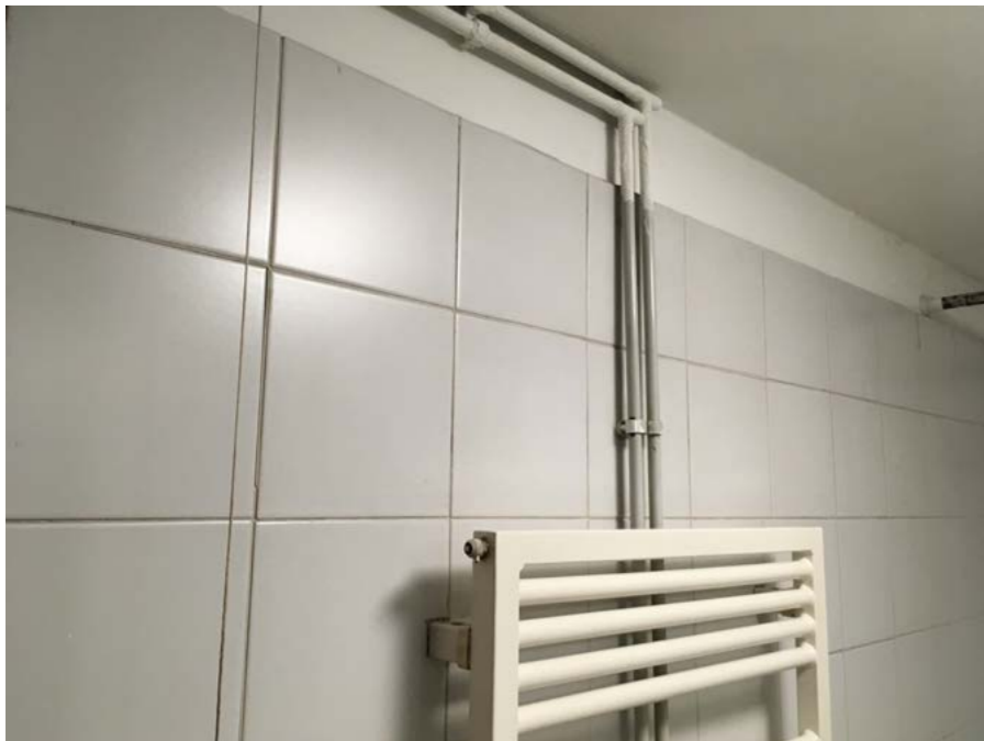
Surface Fixed Pipework from Trench Heater to Non-original Radiator
