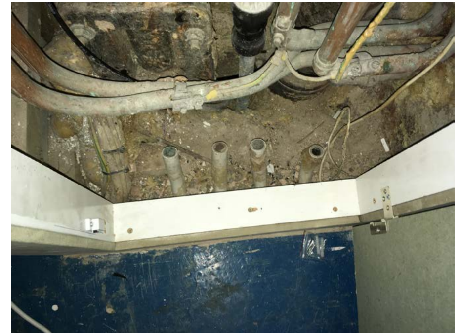
Originally Buried Pipework in 1st Floor Utility Room
