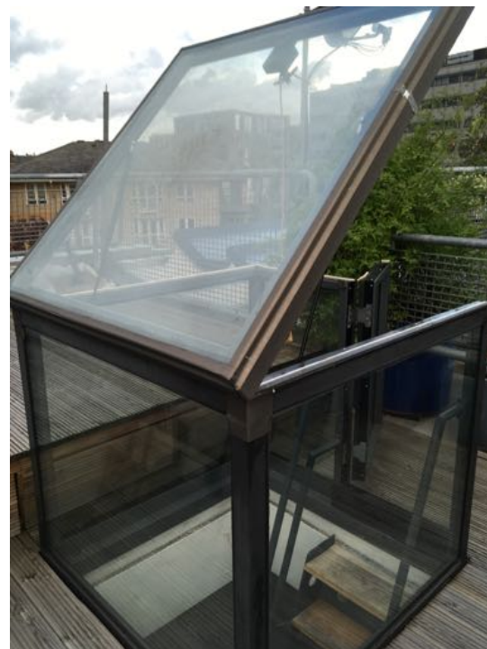
Existing Roof Access Pod
