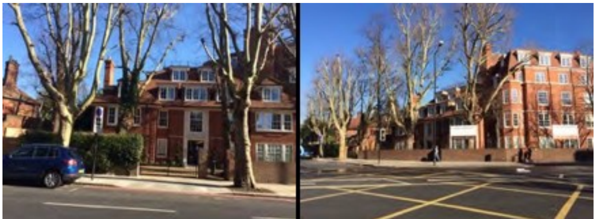
Example of new block of flats viewed from Heath Drive and Finchley Road
