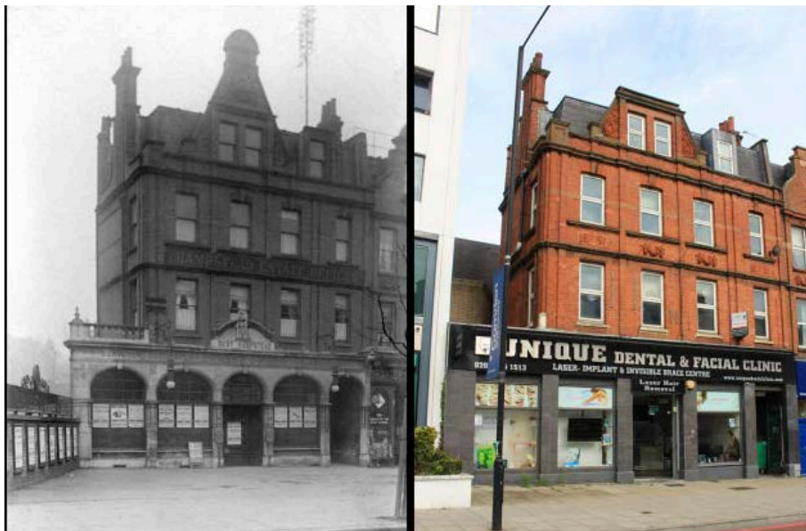
Original and existing shopfronts at 200 Finchley Road
