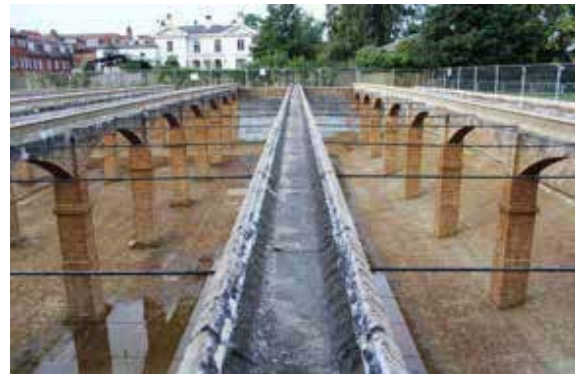
Victorian Engineering Beneath Covered Water Reservoir
