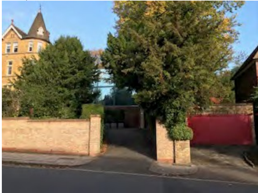
Example of modern infill development
