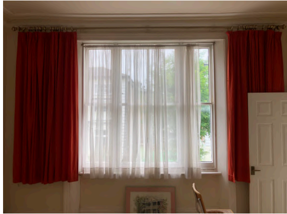
Internal view of triple sash window to front elevation
