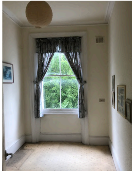
Internal view of single sash window to rear elevation
