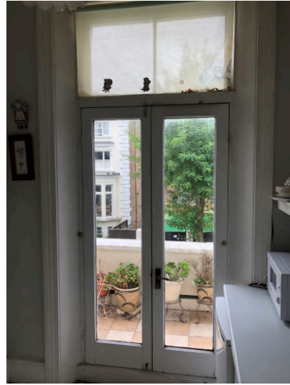
Internal view of French doors to front elevation
