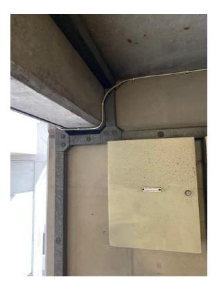
This photo shows the existing 20mm galvanised tube. This will contain the cable to the apartment.
