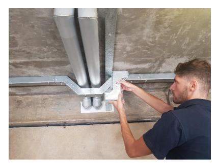
This photo shows the test containment using 45 degree corners going over the pipes entering the apartment.
