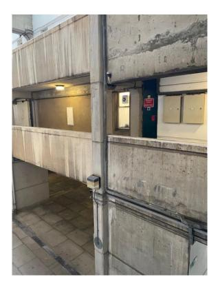
This photo shows how the containment enters the apartments. This will be re used to reduce any disturbance into the apartment.
