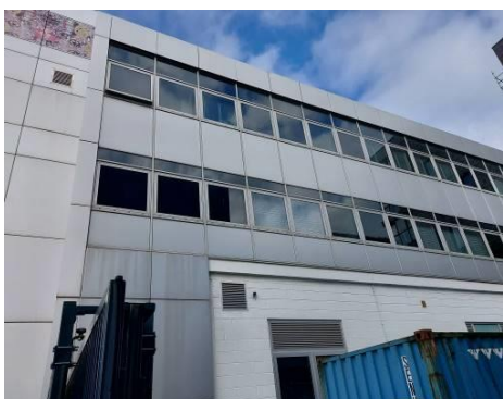
Photograph 1: Eastern elevation of Building 1.
