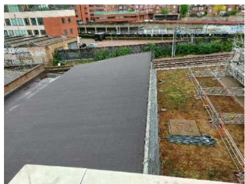
Photograph 5: Roof of Building 2 (left).
