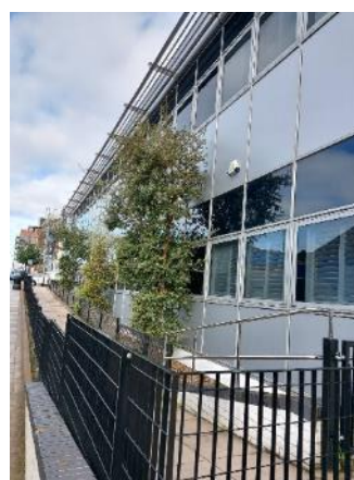
Photograph 8: Southern elevation of Building 1, showing ornamental trees.
