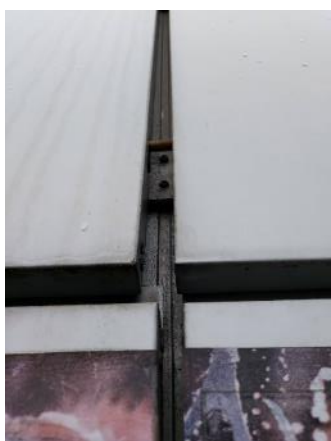
Photograph 7: Example of cladding on Building 1, showing small gaps between and underneath panels.
