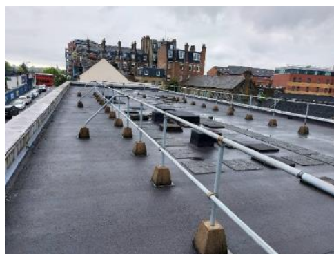
Photograph 6: Roof of Building 1.
