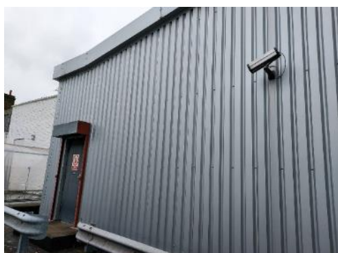
Photograph 3: Exterior of Building 2 (Warehouse).
