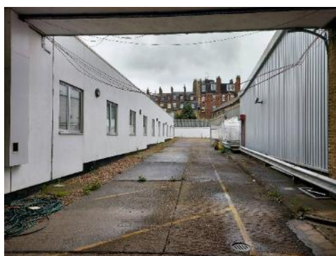
Photograph 4: Undercroft under Building 1.
