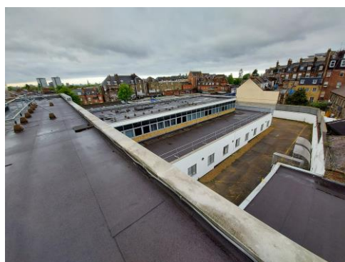
Photograph 2: Roof Sections of Building 1.
