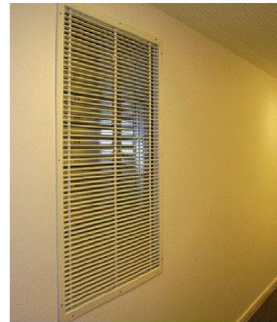
Typical corridor smoke vent grilles
