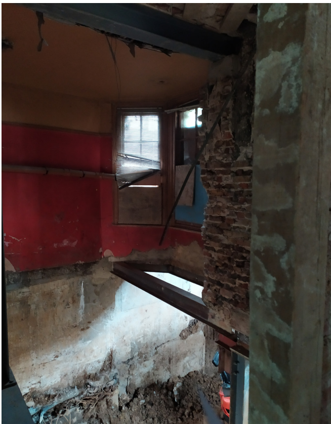
4. Excavated front basement and retained front bow window
