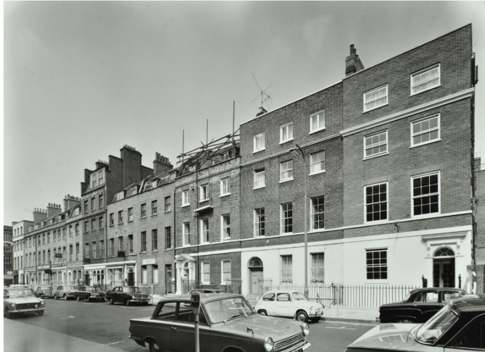
Figure 3: The north side of Percy Street in 1963 (No. 30 has scaffolding on the roof)
