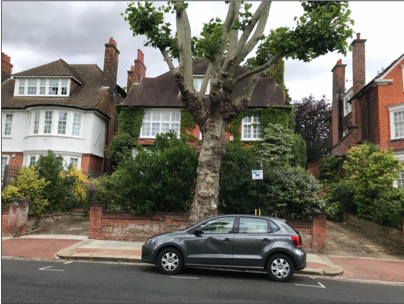
Photograph 2: Frontage of 24 Ferncroft Avenue
