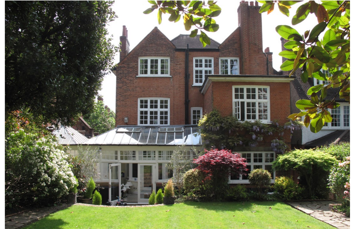
05 - View from the back of garden towards the building and existing steps
