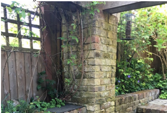
06 - Existing brickwork pier to no.22 side
