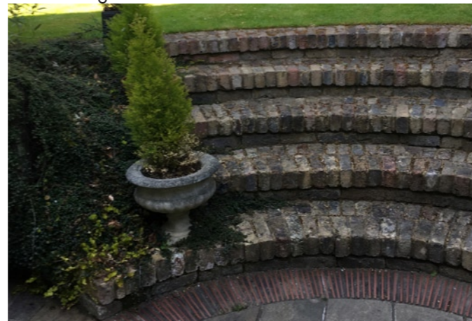
07 - Existing brickwork steps to lawn
