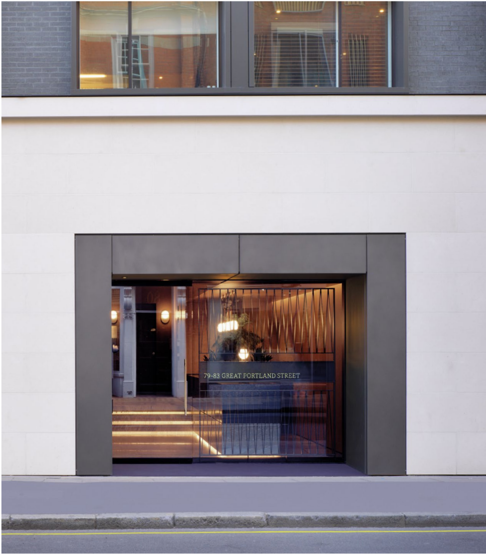
Great Portland Street is a retrofit project where the original 1980's facade has been over-clad in a smooth Limestone and is complimented by the contemporary Adapta Gaelic panels.
