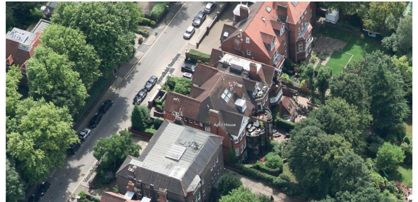
North facing aerial view
