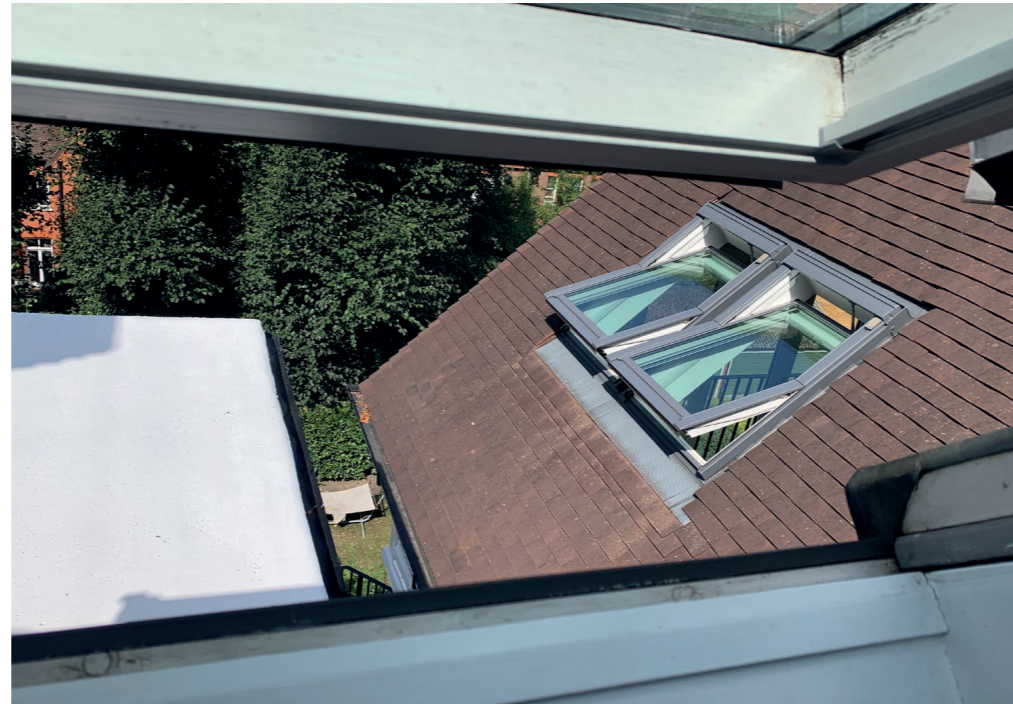
Above, Existing roof lights previously approved.
