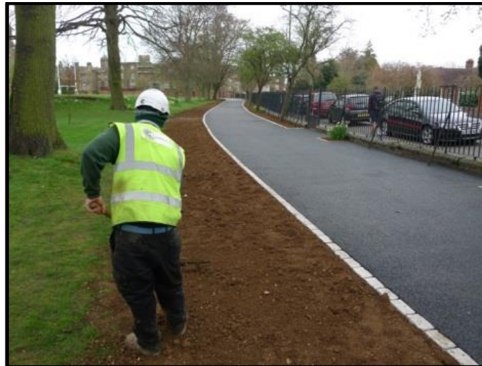
Fig 4 – In the event of 'making good' topsoil will be BS3882 compliant and raked out by hand to no greater depth than 100mm
