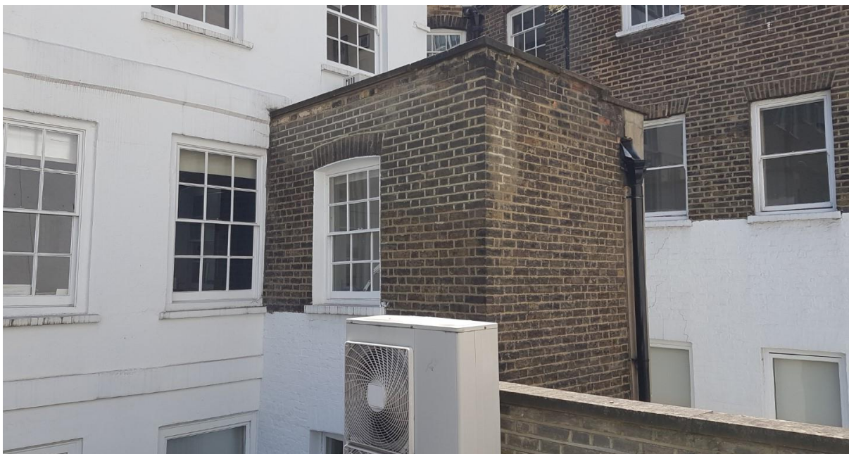
Figure C4 – Photo showing existing condenser unit associated with the Site, noted as 'just audible' at 1 m with other surrounding plant dominant.
