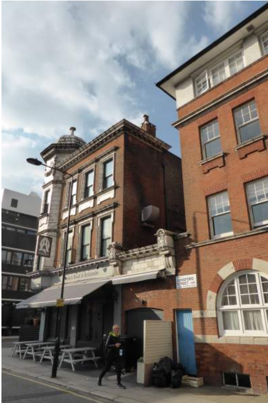
Queens Head and Artichoke Longford Street Elevation
