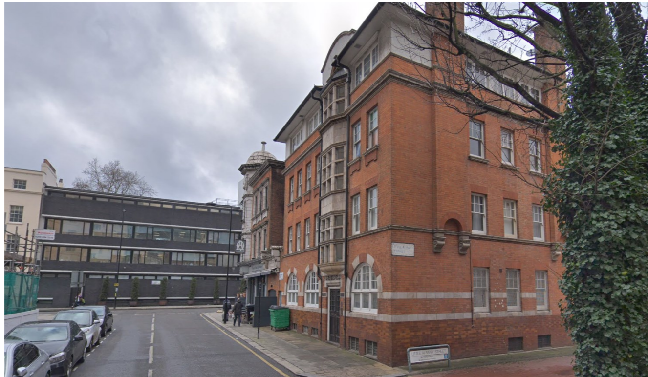
Figure 12: Looking west along the Longford Street.
