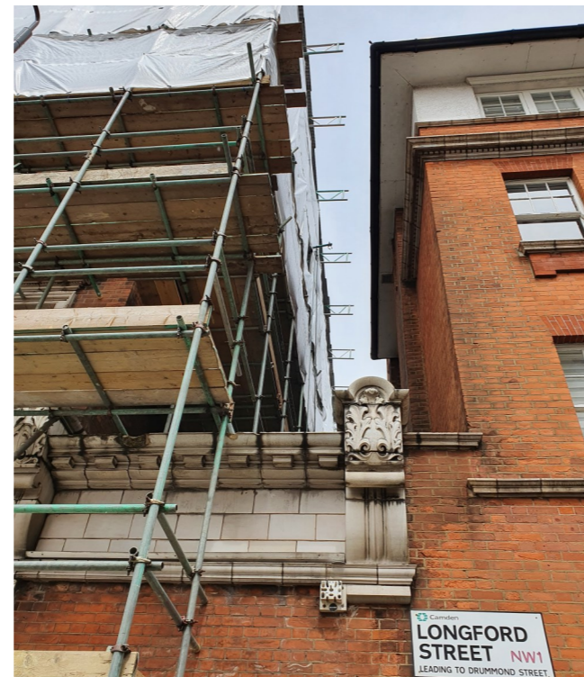
Figure 14: Gap between Nos. 30-32 Albany Street and Walton House.
