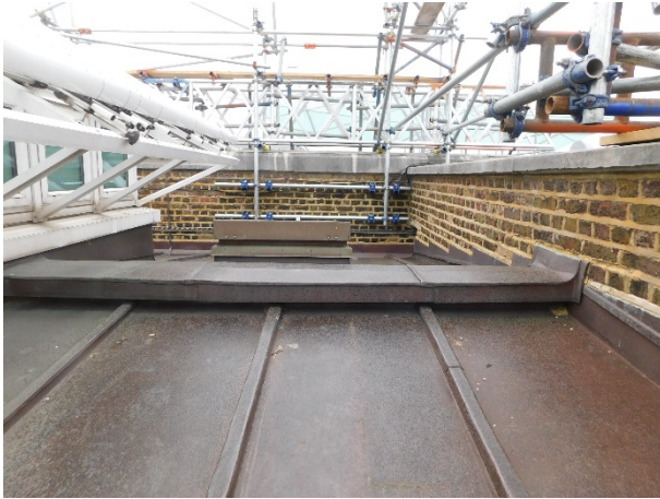
Figure 7: – 2008 ridge detail over G36-37 to be adopted
