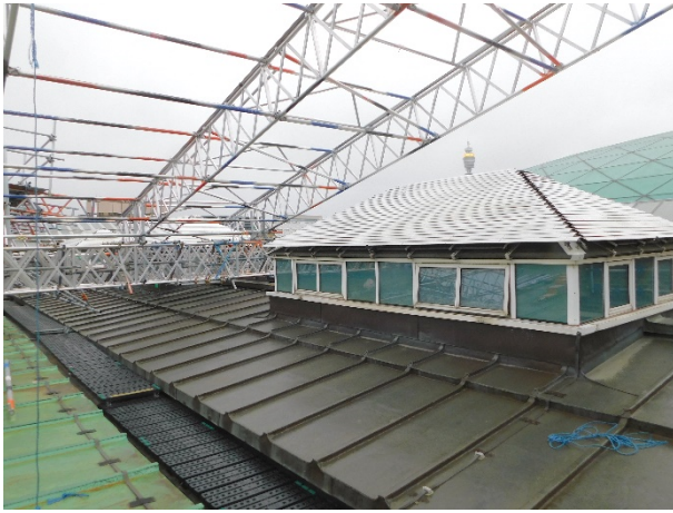
Figure 8:: detail at gutter showing visual impact of raising roof for cross ventilation
