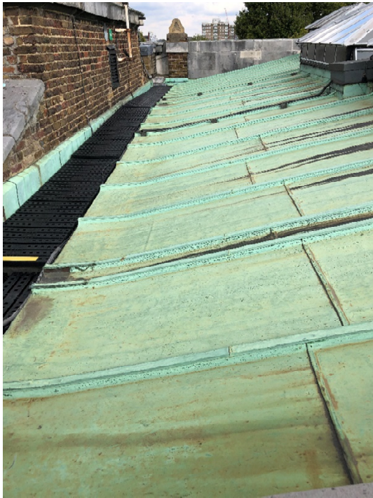
Figure 5: - area of deflected copper roofing
