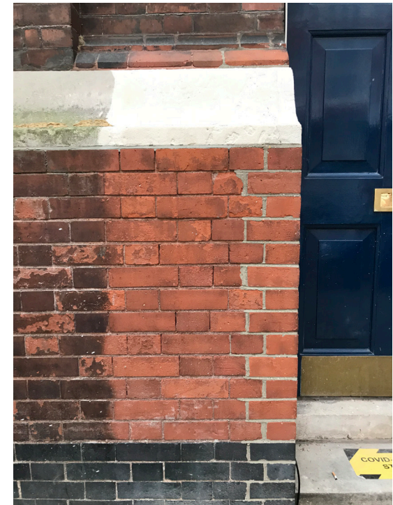
Wet Abrasion Cleaning System: TORC/ JOS
