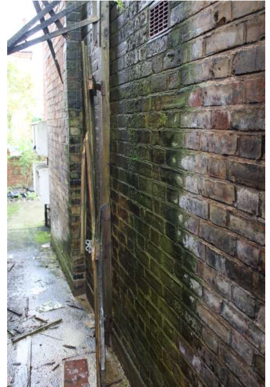
Fig.15. External brickwork showing damp defects
