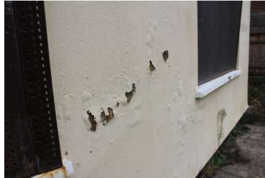
Fig.13. External render showing defects
